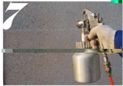
7 喷涂液态花岗石 Spray liquid granite
