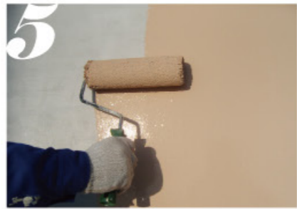
5 涂刷液态花岗石专用中间漆 Brush the special intermediate
